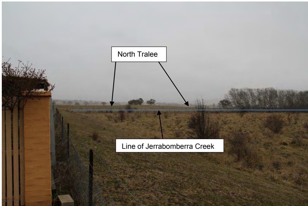
Photograph 1 | View from 36 Bayside Court looking west
